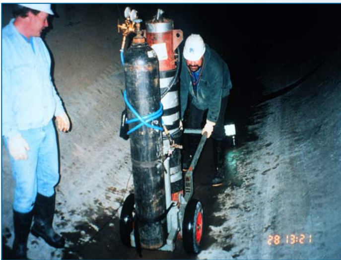
USING HISS HAMMER IN TUNNEL
